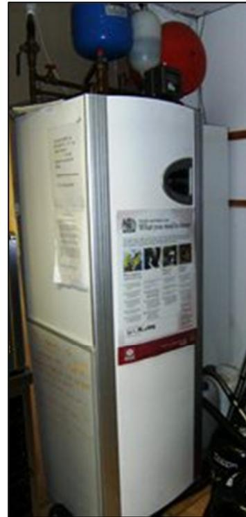
**Picture 1: Ground source heat pump**
